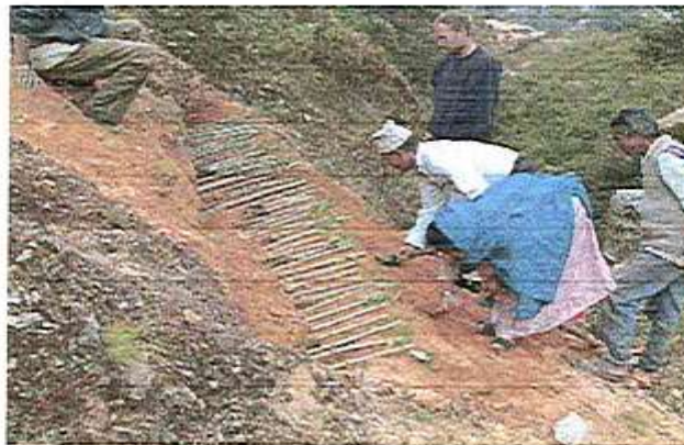
Brush layer construction placing live branch cuttings in slopes
