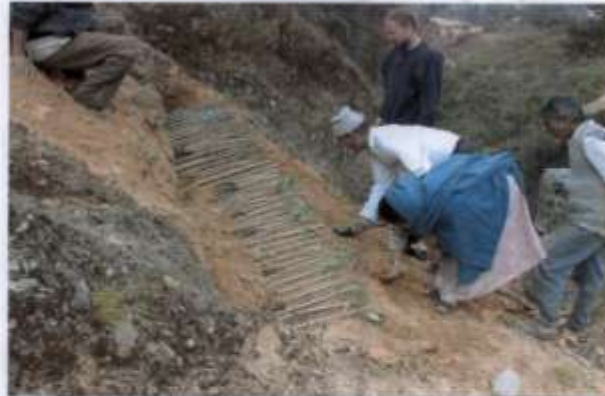
Brush layer construction placing live branch cuttings in slopes
