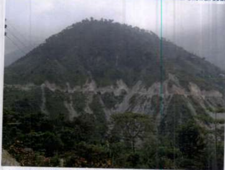
Land Slide on left bank of Kalam Khad due to construction of Banet Road
