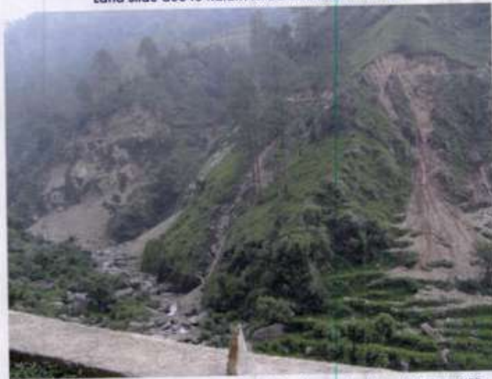
Land Slide on left bank of Kalam Khad due to construction of Kalam HEP
