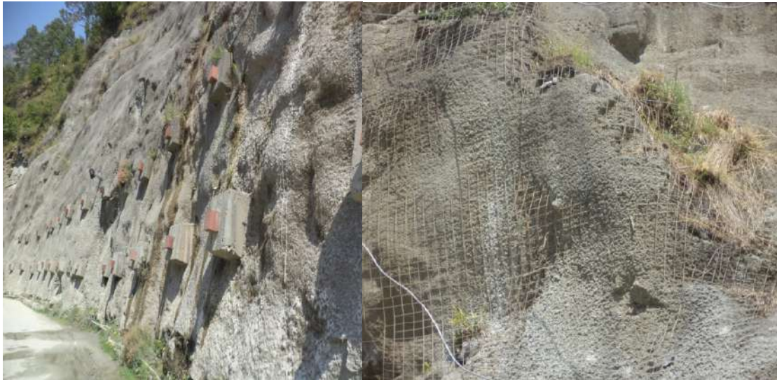
Plate 5.8 – Use of Geo-Jute on Steep Degraded Slopes
