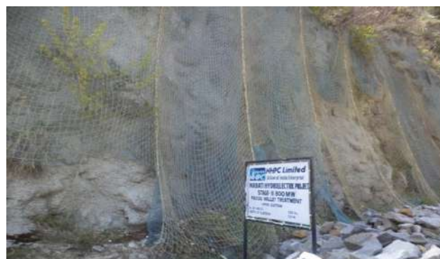
Plate 5.7 – Use of Geo-Jute Mats as Bio-engineering Measure
