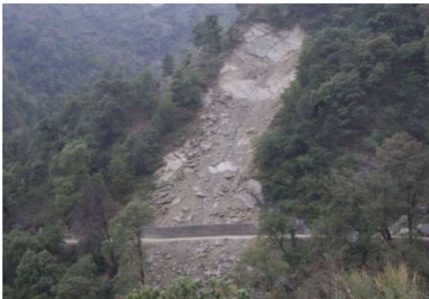
Plate 5.2 – Retaining Wall at the Base of the Landslide to Protect the Road
