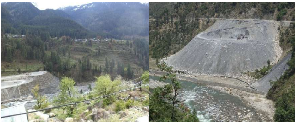
Plate 5.12 - Muck Disposal Sites along the Banks of the Sainj River
