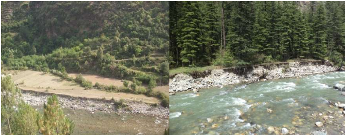
Plate 5.11 - Need of Retaining Wall Construction to Protect the River Bank from Soil Erosion
