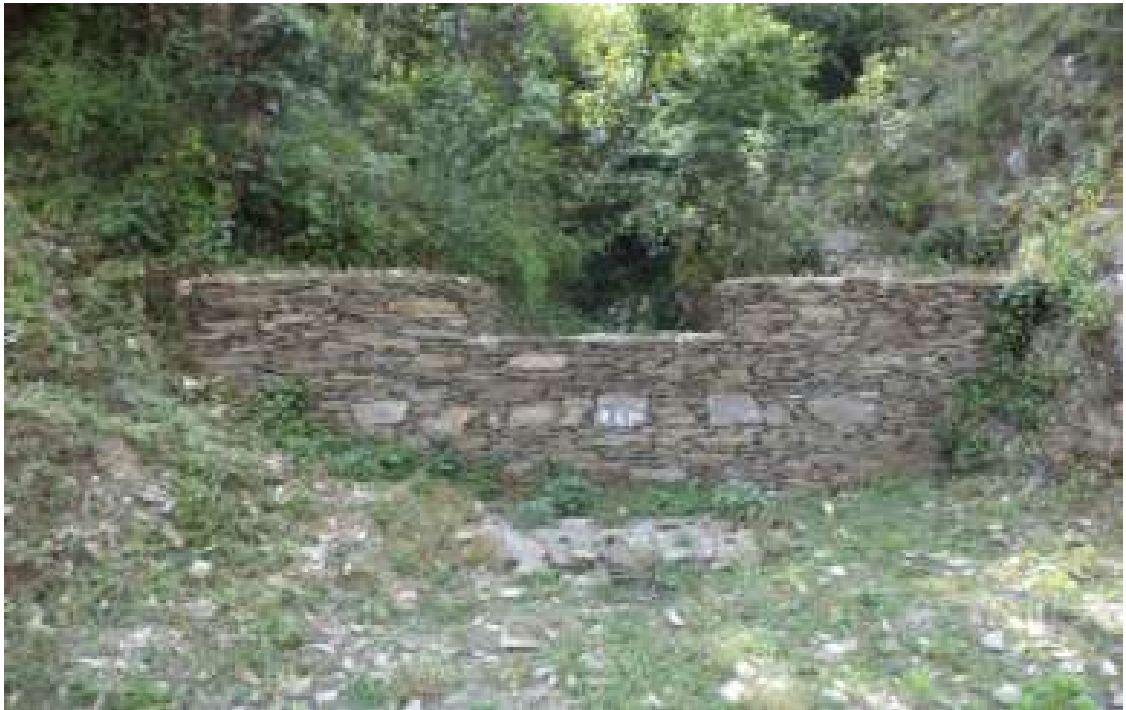
Plate 5.10 –Typical Dry Stone Structure Made of Slate Type Stones is More Stable
